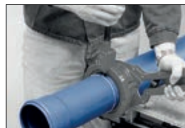
Cutting to length with a cutting and chamfering tool (FIGURE 16)
