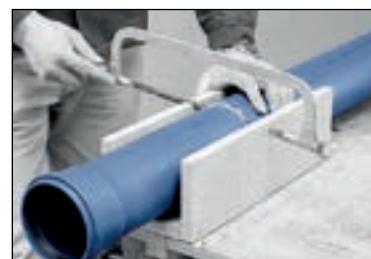
Cutting to length with a fine-toothed saw (FIGURE 17)
